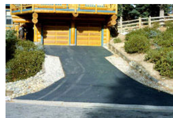
Residential BMPs include slotted drains, drywells, retaining walls, and use of native vegetation or mulch to stabilize slopes or eroding areas.
